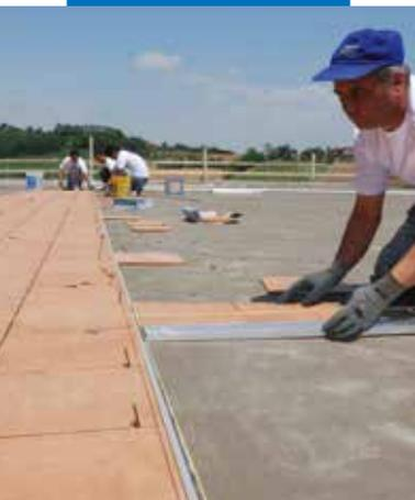
Installing ceramic with Kerabond + Isolastic
