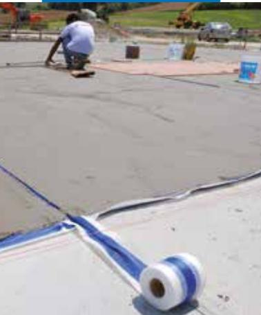
Waterproofing screeds with Mapelastic and Mapeband
